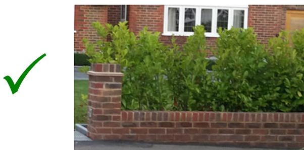
Where the need for enclosure is a requirement, front boundary walls and gates should not exceed the height allowed under Permitted Development Rights (maximum 1m high within 2m of the front boundary).
