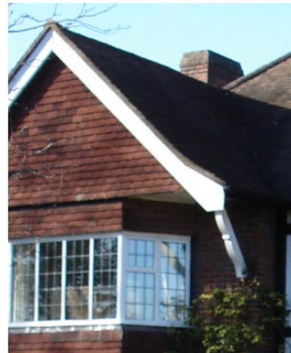
When refurbishing, replacing or extending the roof, existing chimneys should be retained.
