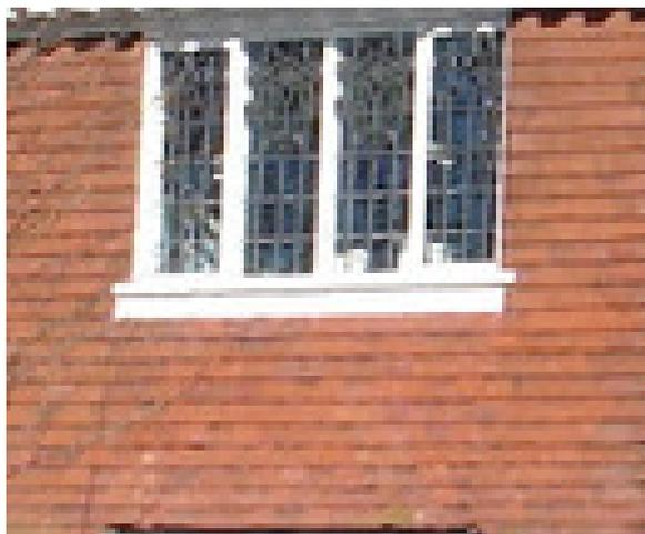
Tile hung first floor elevations or bays with tiles to match the main roof are also typical features.
